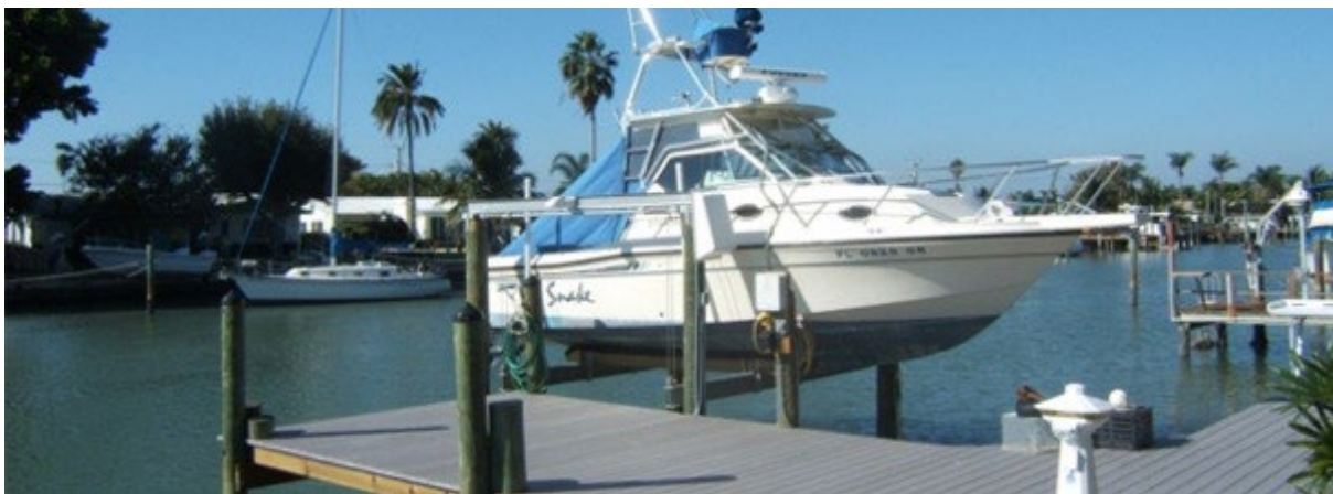
Figure 3.13: Example of a boat lift and fixed jetty structure.
