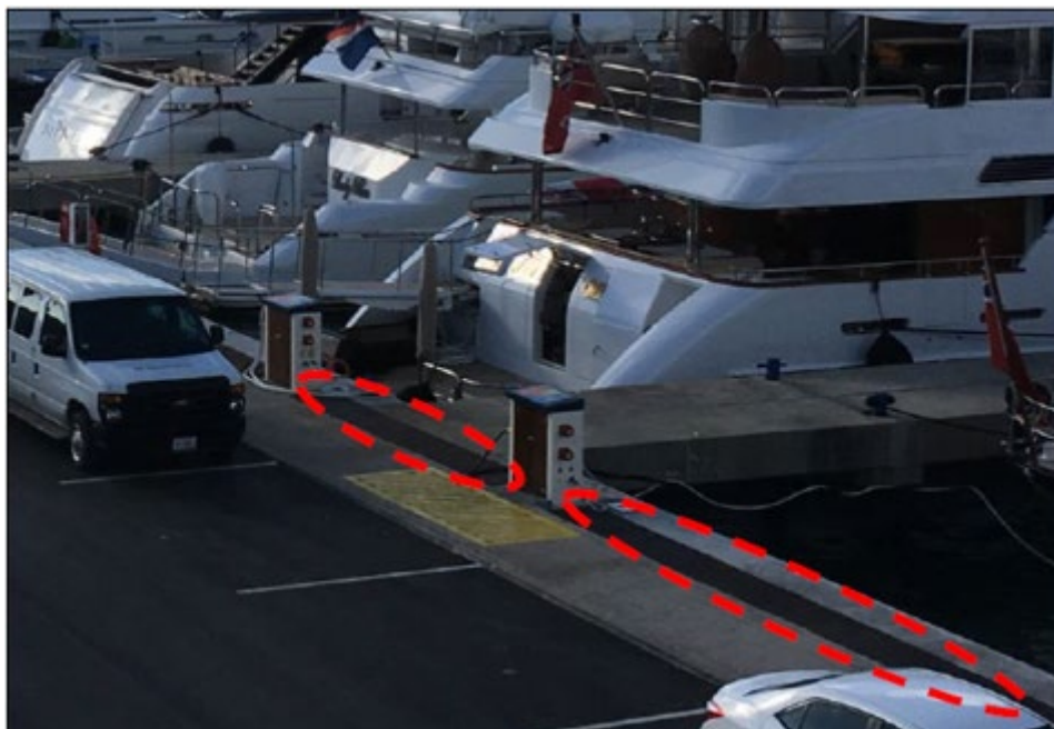
Figure 3.16: Pre-installed ducts and pedestals for water and electricity
