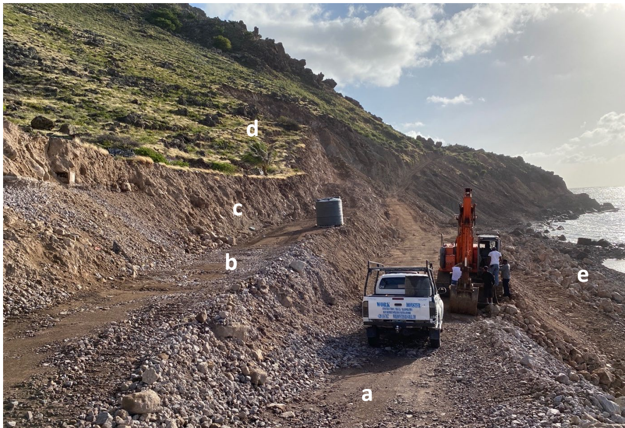
Figure 5.7: Section 2: Existing unpaved road (a), safety bench (b), hillside profiling (c). (d): part of the vegetation that still needs to be cleared. In the right part of the picture, near the shore line, the construction of the rock revetment is visible (e).
